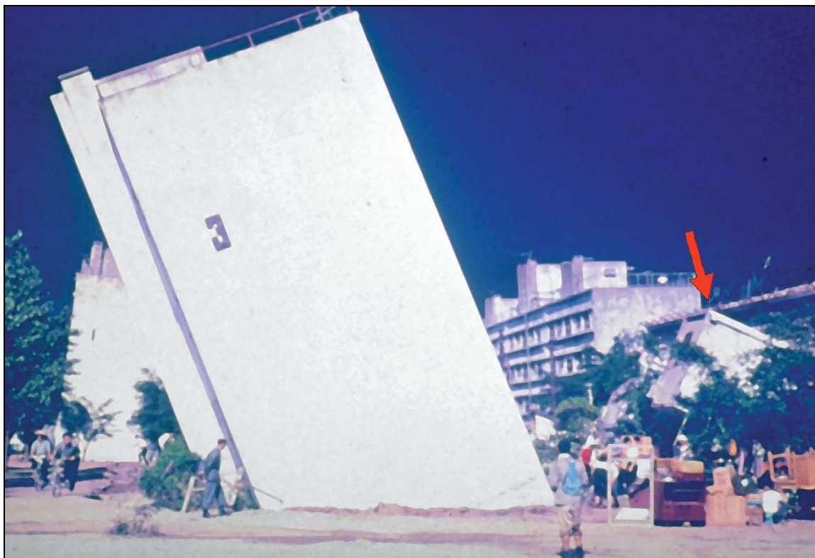
Figure 102: Sinking Buildings. During the above earthquake, building number 3 sank and tipped 22 degrees as the ground partially liquefied. Another building, seen at the red arrow, tipped almost 70 degrees, making its roof nearly vertical.
