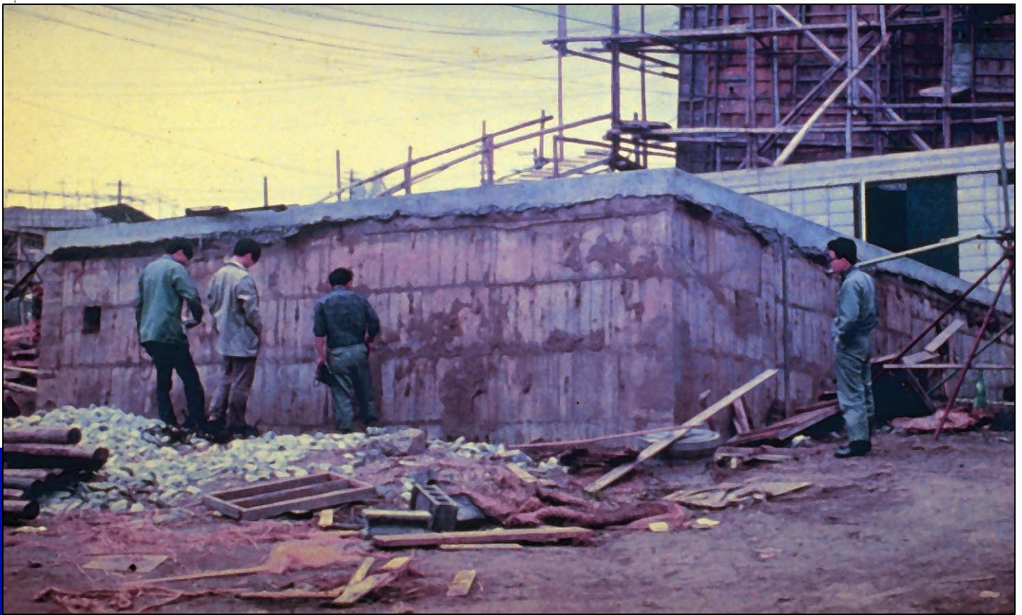
Figure 101: Floating Tank. During a 1964 earthquake in Niigata (NEE-gat-ah), Japan, the ground turned to a dense liquidlike substance, causing this empty concrete tank to float up from just below ground level. This was the first time geologists identified the phenomenon of liquefaction , which had undoubtedly occurred in other large earthquakes. Liquefaction has even lifted empty tanks up through asphalt pavement 1 and raised pipelines and logs out of the ground. 2 In other words, buried objects less dense than surrounding soil rise buoyantly when that soil liquefies. What causes liquefaction? What would happen to buried animals and plants in temporarily liquefied sediments?
