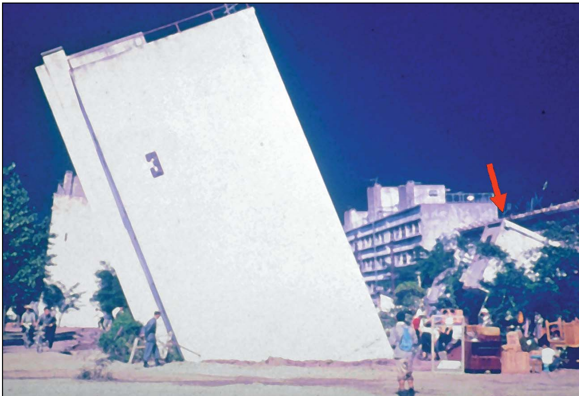
Figure 31: Sinking Buildings. During the above earthquake, building number 3 sank and tipped 22 degrees as the ground partially liquefied. Another building, seen at the red arrow, tipped almost 70 degrees, making its roof nearly vertical.
